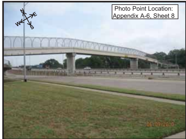
Photograph 28. Pedestrian Bridge at IH 45 and Lenway, from the southbound frontage road, looking northbound.
