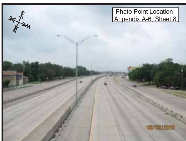
Photograph 32. IH 45 and Lenway, taken from the pedestrian bridge, looking south on IH 45
