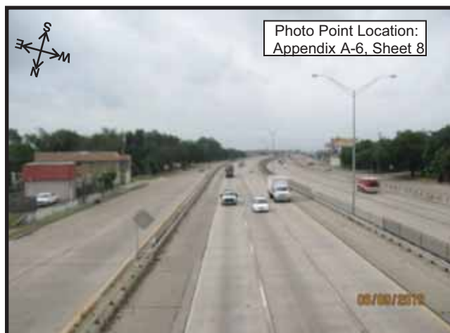
Photograph 34. IH 45 and Lenway, from the pedestrian bridge, looking south on IH 45
