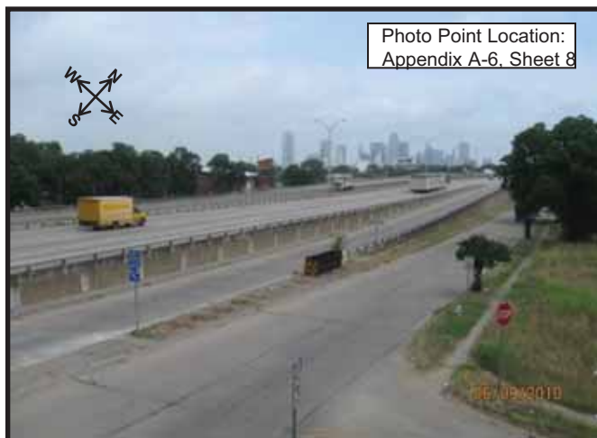
Photograph 35. IH 45 and Lenway, from the pedestrian bridge ramp on the northbound frontage road, looking northwest
