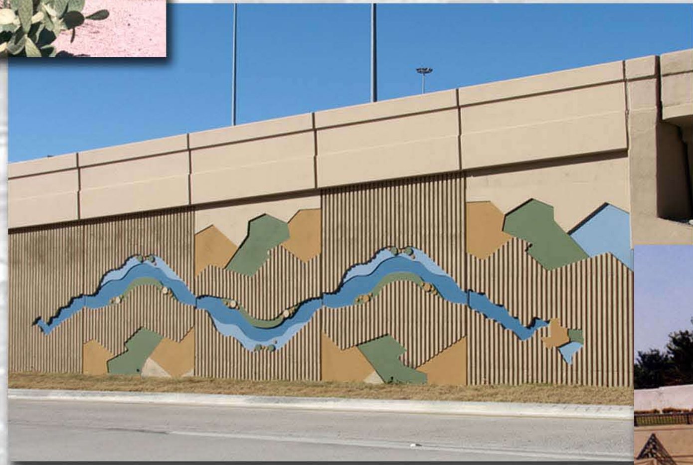
FORM LINE CONCRETE
